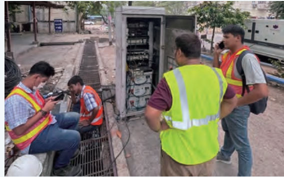
Huawei's team immediately rushed to restore communications services after an earthquake in Myanmar.
